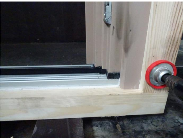
Picture 11 Frame connection to threshold, seen from inside
