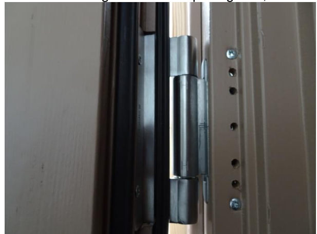
Picture 6 Hinge seen from rebate, at top
