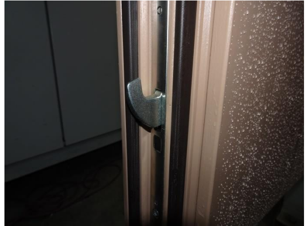
Picture 20 Auxiliary lock
