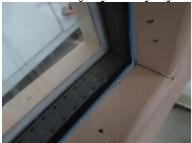
Picture 18 Sealing of glazing, seen from outside
