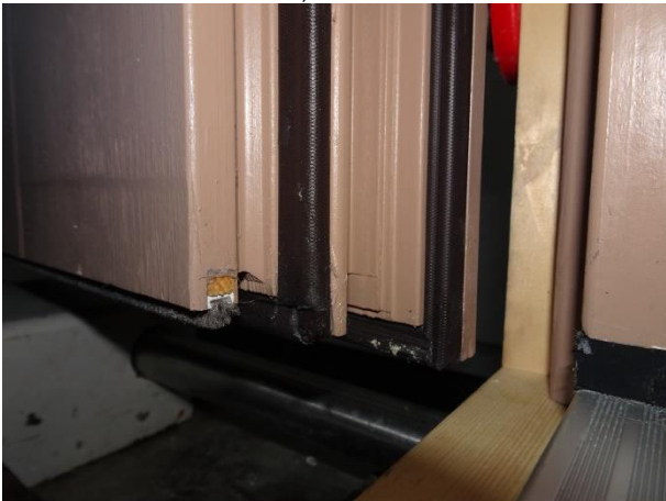
Picture 15 Leaf seal at bottom
