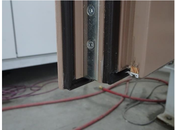
Picture 14 Leaf seal at bottom
