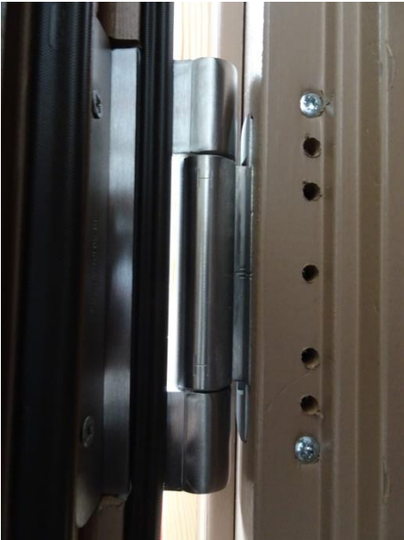
Picture 7 Hinge seen from rebate, at centre
