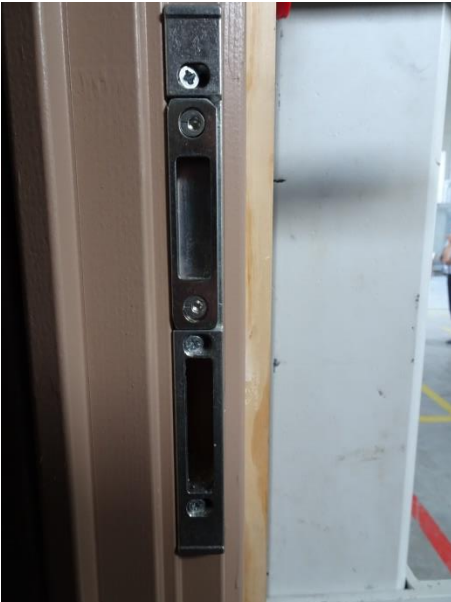
Picture 21 Strike plate for main lock
