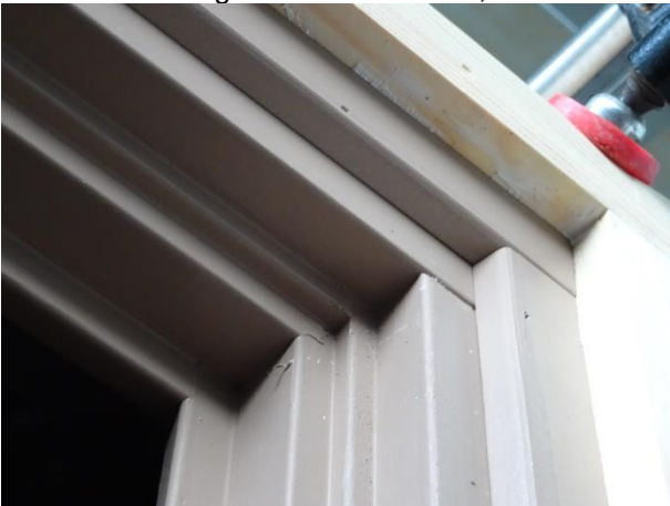
Picture 9 Frame at top, corner design, seen from inside
