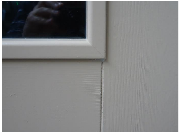
Picture 16 Internal glazing bead and glazing corner
