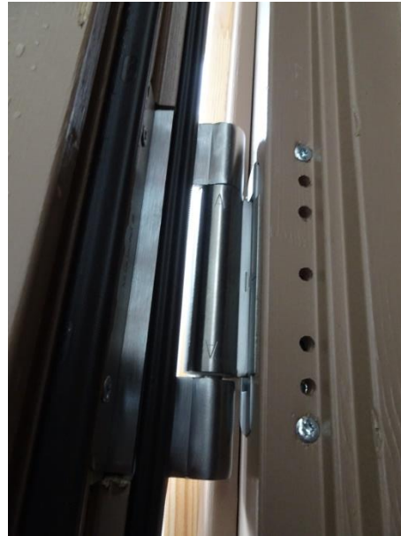
Picture 8 Hinge seen from rebate, at bottom
