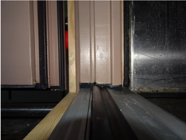
Picture 13 Threshold, seen from rebate
