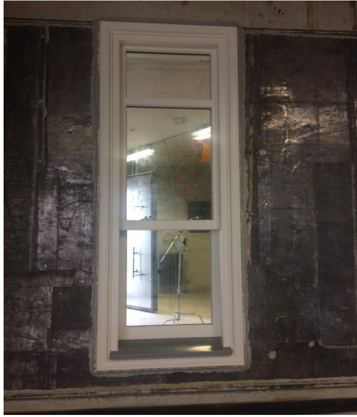
Resim No. 1 Monte Deneş Numunesi / Photo No.1 Mounted Test Specimen
